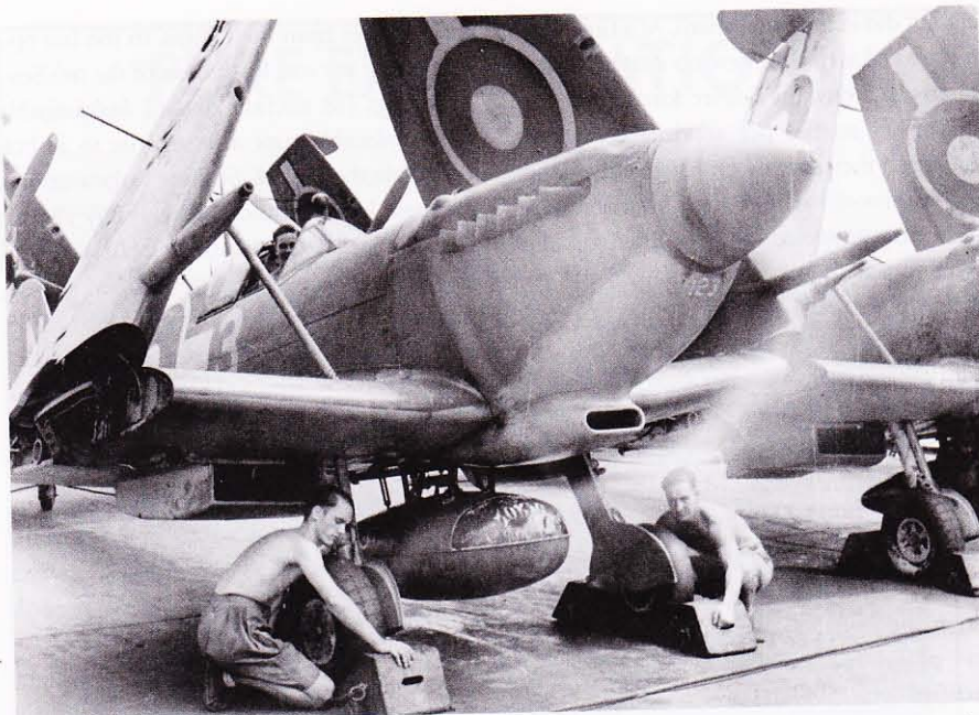
A Seafire III of No. 38 Naval Fighter Wing warms up onboard Implacable in mid-1945. Note the Curtiss P-40 drop tank, which proved more reliable than the 90-gallon slipper tank.
